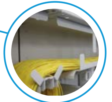
Cable raceways for horizontal communication between adjacent distribution frames
