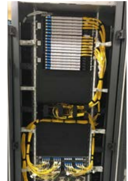
3U Horizontal Overlength Storage integrated in 19" frame
